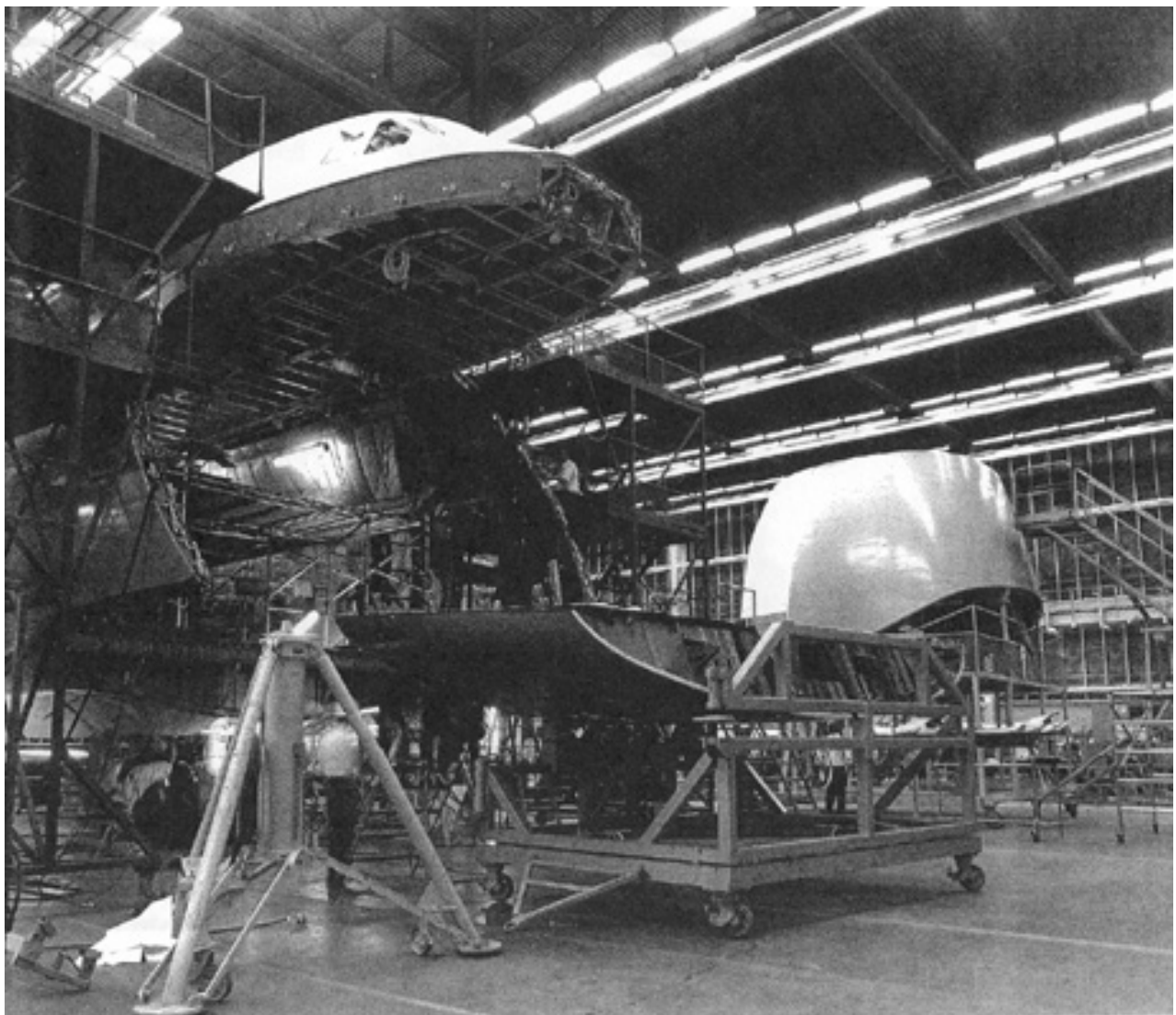
The gaping cargo compartment of a C-5A during nose assembly, February 1968.
