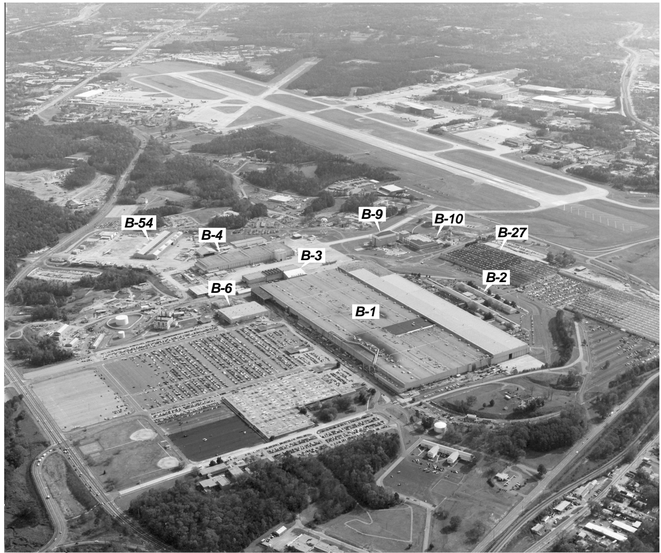
Aerial view of Air Force Plant 6, ca. 1990.
