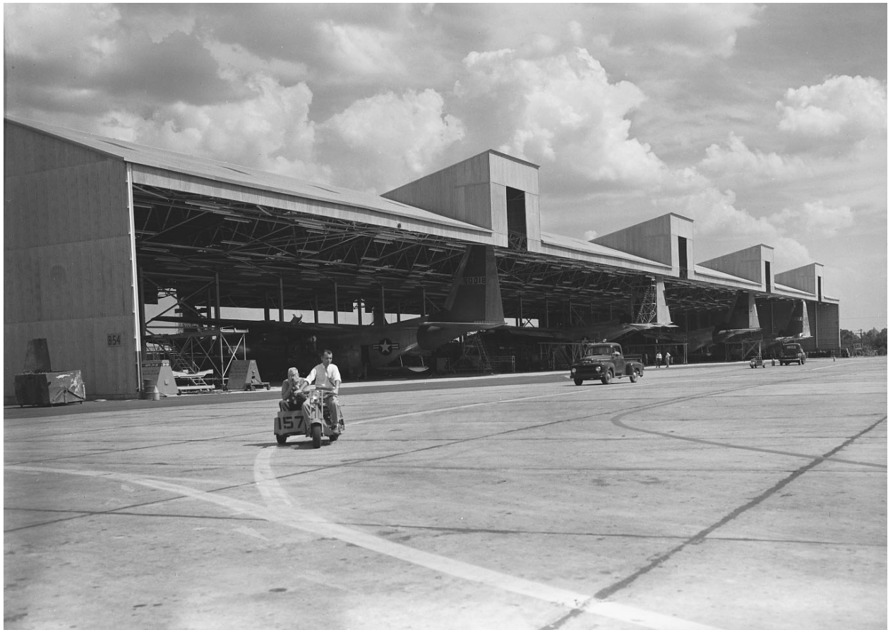
Eight-plane modification hangar, B-54, ca. 1958.
