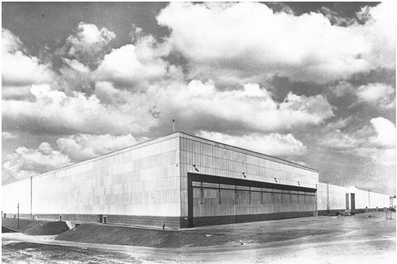
Main assembly building (B-1) at Air Force Plant 6. This view, taken shortly after completion in 1943, is of the southeast corner of the building, showing the high-roof of the main assembly bay, the hangar doors, and the entrance to Tunnel 5 (lower left). Manufacturing activities were conducted on the ground floor and the two mezzanine sections. The basement contained cafeterias, locker rooms, offices, tool cribs, and room for temperature control and air compressing machines. The tunnels in the basement were used by motor vehicles and for employees entering or leaving the building through head houses located near the parking lot on the north side of the factory.
