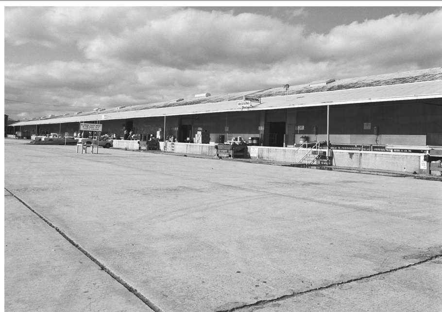
B-27, Material and Fabrication Building, November 1986.
