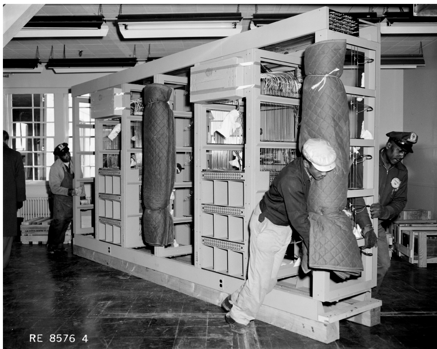
New analog computer being installed in Engineering, northeast wing of B-2 building, January 1958. An opening had to be cut over the door to get the machine in the building.
