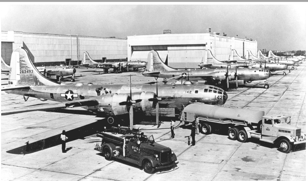
Newly completed B-29 aircraft are serviced on the tarmac outside the paint shop (B-3, in background), ca. 1944.
