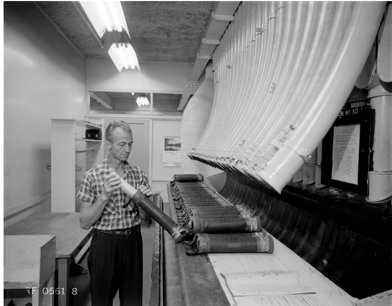
A system of pneumatic tubes carried mail through B-1 building, 1958.
