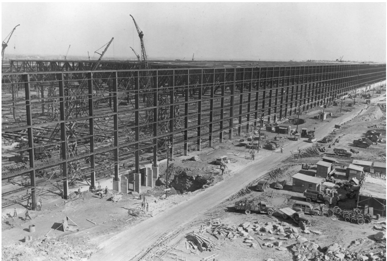
The main assembly building (B-1) under construction, November 1942.
